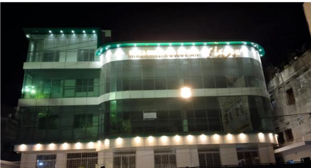
Pic 1: College building with Greene and LED's
