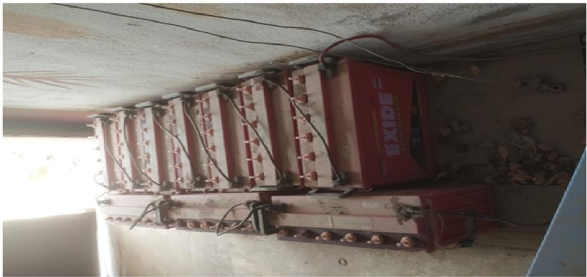
Pic-2 Installation of solar cell on the roof and related batteries
